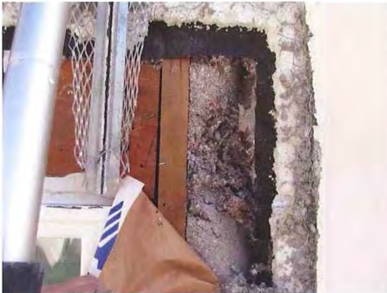
May 14, 2019, Disc IT3, Photograph 52, JBF, south elevation of Building B - Unit 3104, open stud framing with no exterior sheathing.
