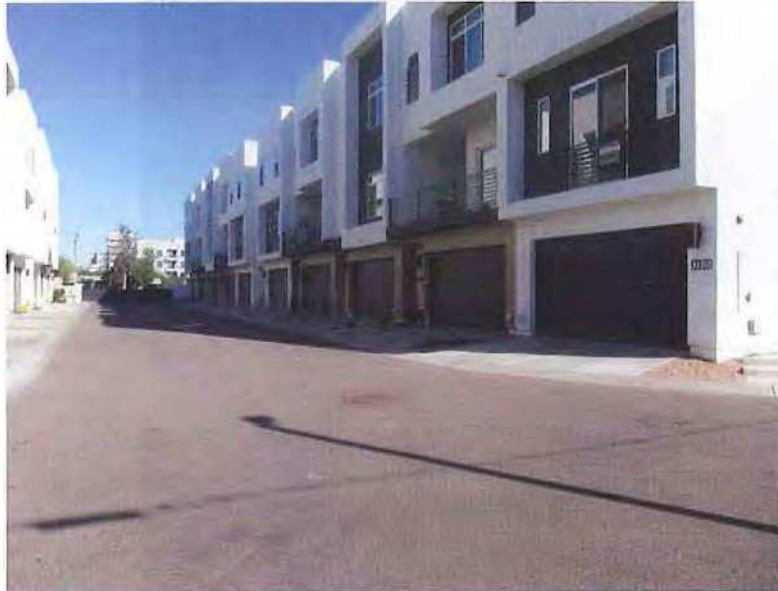
December 19, 2018, Photo 14, OBS1, JBF, overview of the elevation showing limited panel size available for LFRS.
