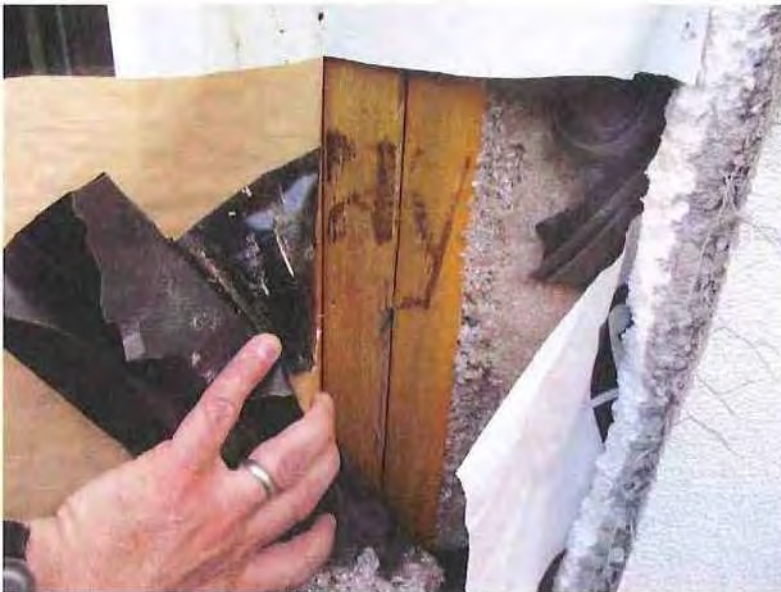
May 13, 2019, Disc II1, Photograph 156, JBF, south elevation of Building C - Unit 3117, open stud framing with no exterior sheathing.
