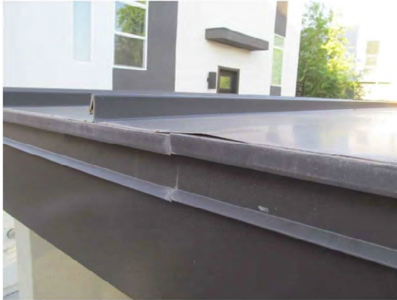
August 23, 2021, Disc OBS8, Photograph 18, JJF, pool cabana, unsealed and bulging edge.
