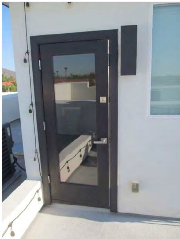
August 23, 2021, Disc OBS8, Photograph 23, JJF, Unit 3106, overview of roof access door.
