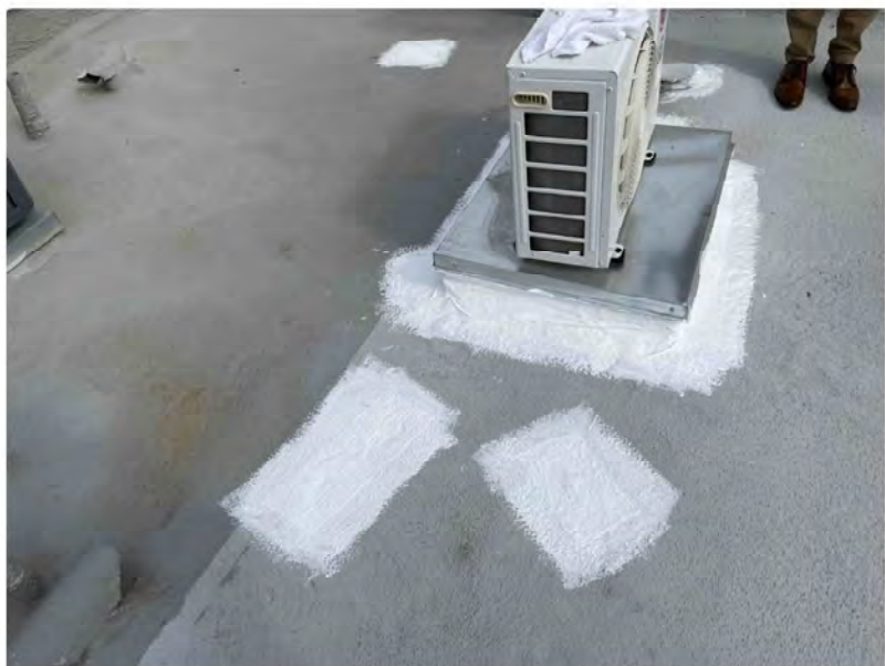
Nautilus-provided photograph, Bates Number GALLERY-NBC_005059, Unit 3112, Nautilus roof repair.
