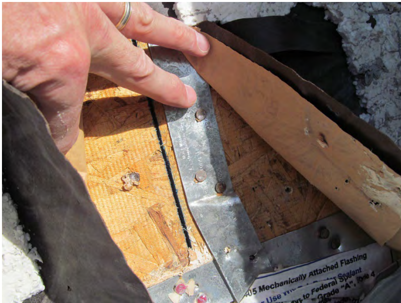
Building B – Rear Elevation, 177D Disc IT5
