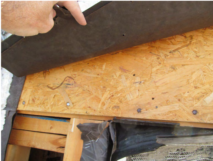
Building D – Rear Elevation, 130F Disc IT7
