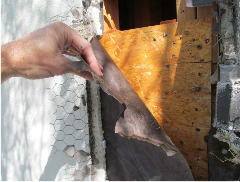
Building D – Rear Elevation, 88F Disc IT7
