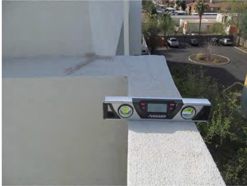
March 11, 2021, Disc IT10, Photograph 70, SSR, Building A, roof parapet wall slopes 6-percent outward.
