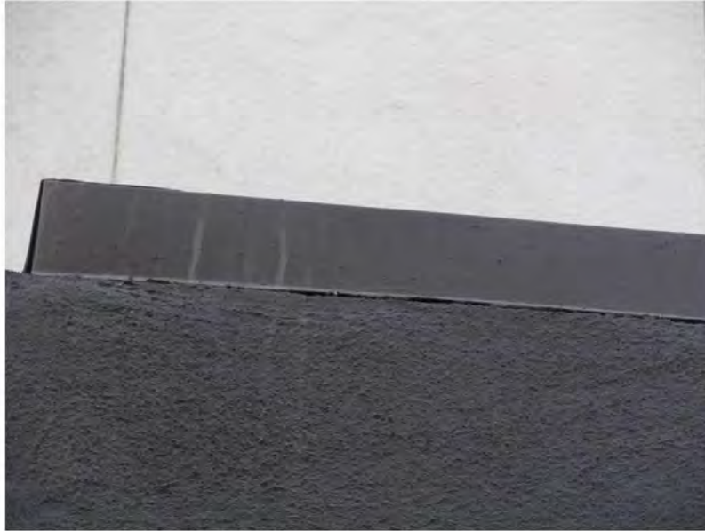
March 10, 2021, Disc OBS5, Photograph 69, SSR, Building. B, awning edge flashing inset at stucco.
