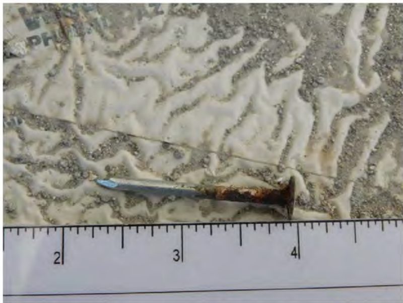
March 10, 2021, Disc IT9, Photograph 188, PER, Building C, holes and stains in Xtraflash SAM allow moisture intrusion.
