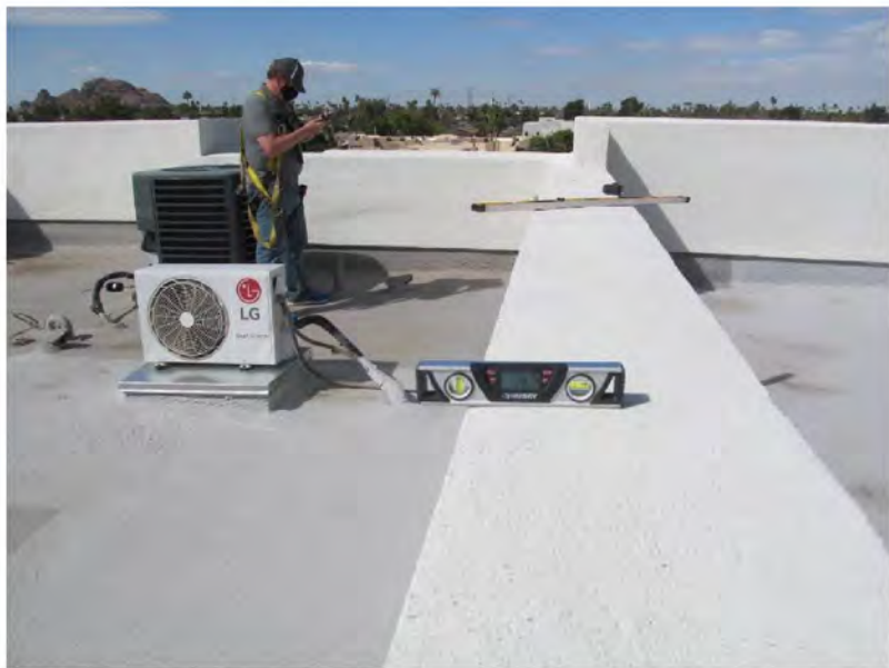
March 11, 2021, Disc IT10, Photograph 227, SSR, Building A, roof parapet wall slopes 2-percent.
