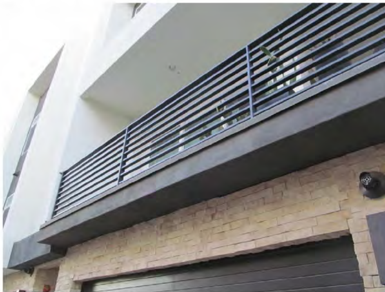
March 10, 2021, Disc OBS5, Photograph 77, SSR, Building B, deck edge flashing correctly installed at stucco.
