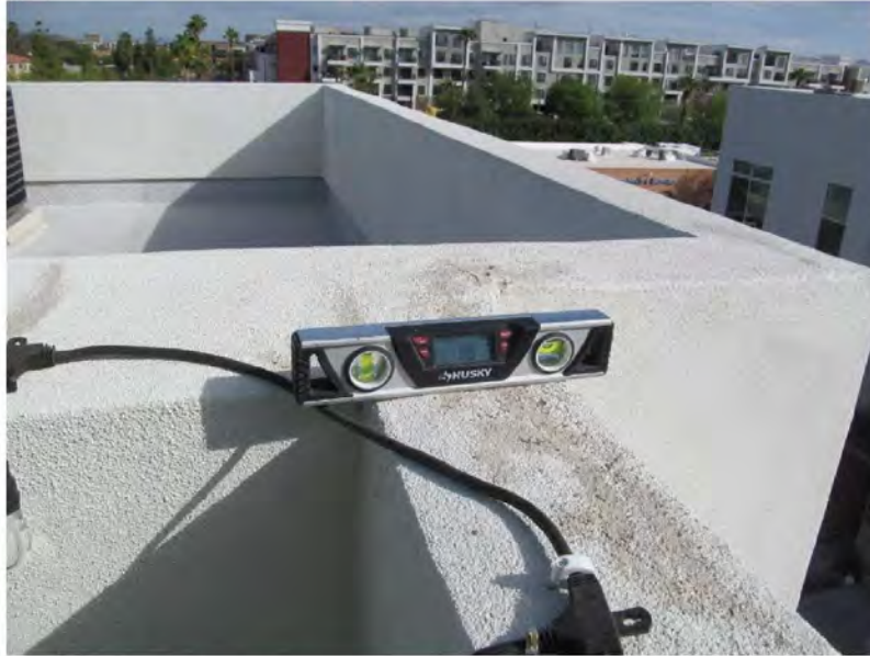
March 11, 2021, Disc IT10, Photograph 76, SSR, Building A, roof parapet wall slopes 0.8-percent inward.
