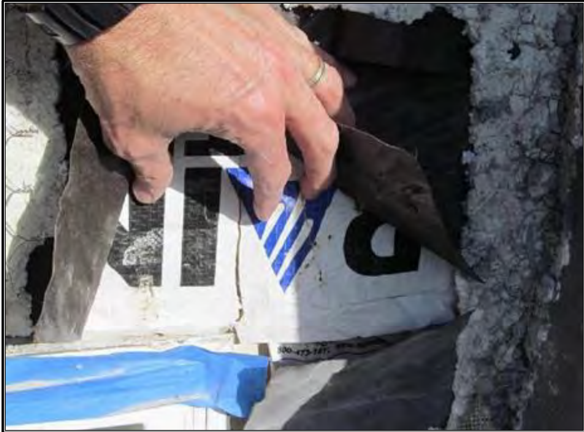
Photo #3 (Pltff Photo Disc ITS Photo 178): One layer of WRB over sheathing.
