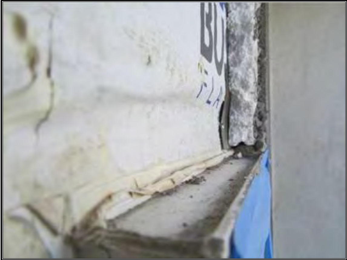
Photo #1 (Pltff Photo Disc IT6 Photo 280): Window head exposed during DT.
