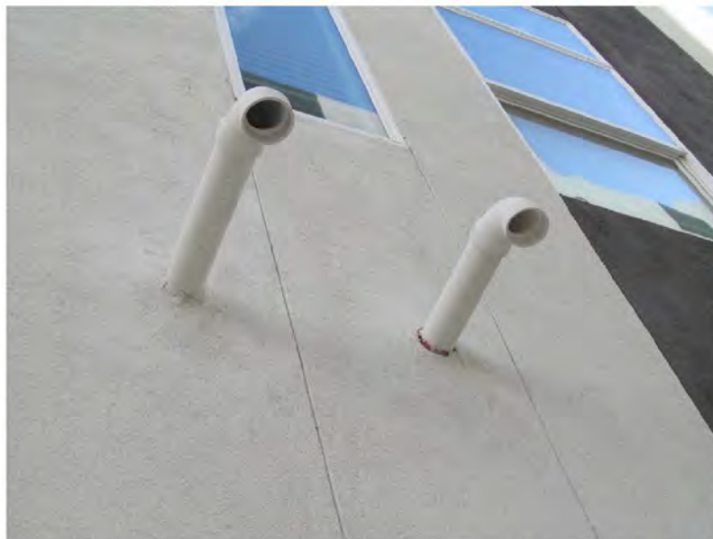
March 11, 2021, Disc OBS 6, Photograph 30, JJF, Building C, vertical control joints were provided on side elevations at re-entrant corners.
