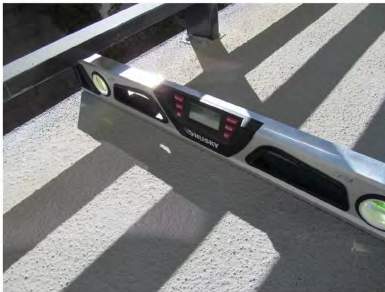
October 15, 2019, Disc OBS3, Photograph 36, SSR, Building C - Unit 3123, 1.4-percent slope at the deck edge.
