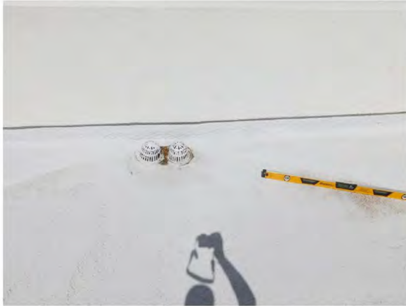
March 11, 2021, Disc OBS7, Photograph 361, PER, Building C, 0-inch-per-foot slope at cricket towards point of drainage.
