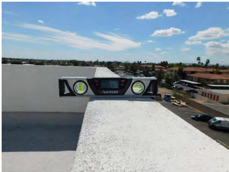
March 11, 2021, Disc OBS7, Photograph 289, PER, Building D, roof parapet wall slopes 3.3-percent inward.
