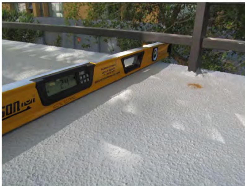
March 10, 2021, Disc IT8, Photograph 351, SSR, Building A - Unit 3124, deck perimeter flashing 2.4-percent slope.
