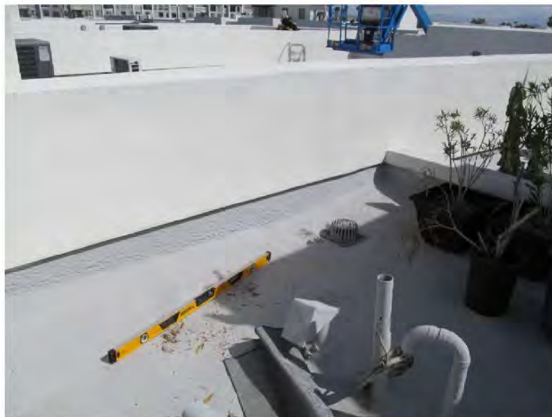
March 11, 2021, Disc OBS7, Photograph 293, PER, Building D, 0-inch-per-foot slope at cricket towards point of drainage.
