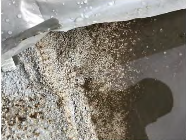
Nautilus-disclosed photo, disclosed on June 16, 2021, Building B – Unit 3110, Photo Number 14, ponding water at roof.
