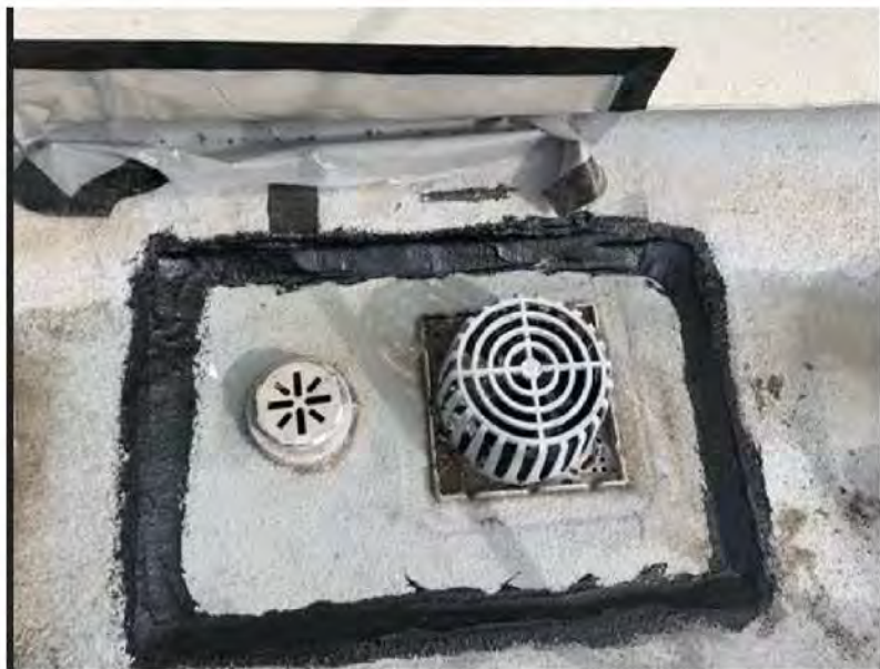
Nautilus photo, disclosed on June 16, 2021, Building B – Unit 3110, Photo Number 21, temporary repairs to reduce future roof leaks.
