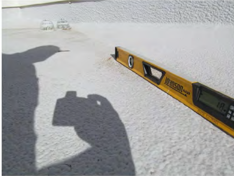
March 11, 2021, Disc IT10, Photograph 49, SSR, Building A, 1/8-inch-per-foot slope at cricket towards point of drainage.
