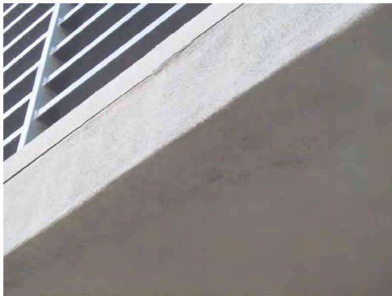
March 11, 2021, Disc OBS6, Photograph 58, JJF, Building C, deck edge flashing inset at stucco.
