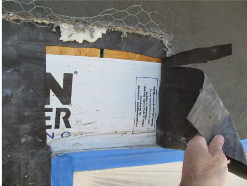
March 10, 2021, Disc IT7, Photograph 136, JJF, Building D, one layer of WRB over sheathing.
