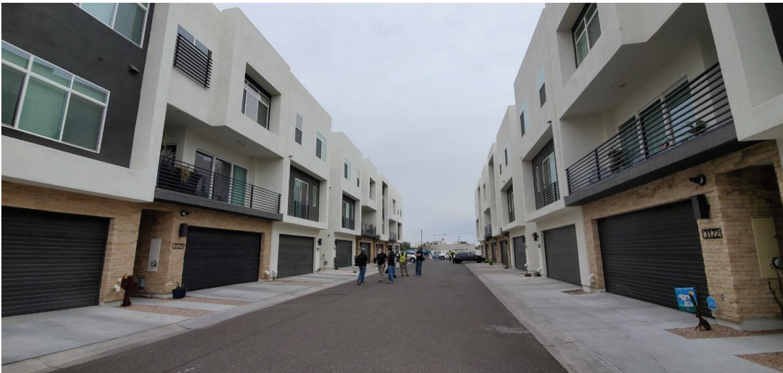
Front elevation of the four buildings (two building in foreground, two buildings in background).
