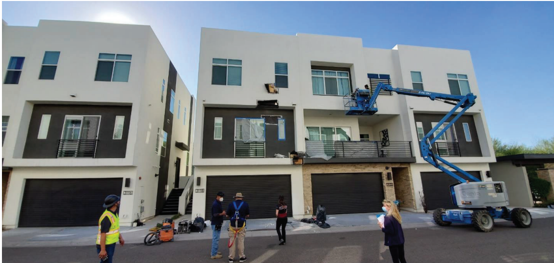
Typical view of destructive investigation work in-progress.
