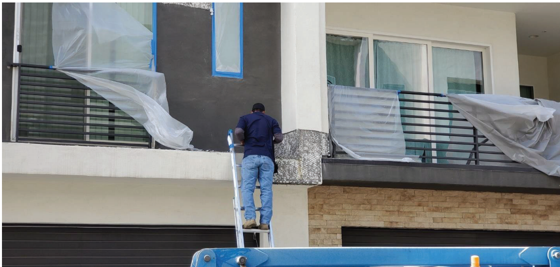
Typical view of destructive investigation work through the stucco cladding.
