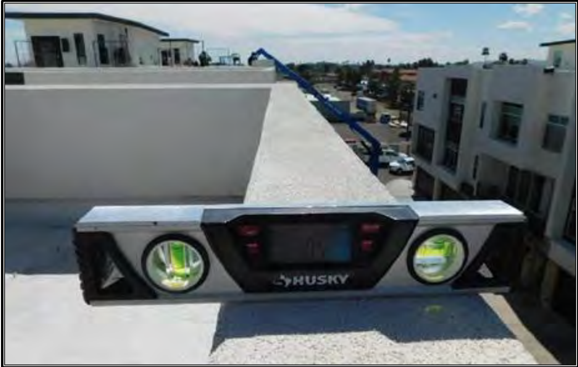
Photo #5 (Pltff Photo Disc OBS7 Photo 350): Roof parapet wall 0.5% slope.
