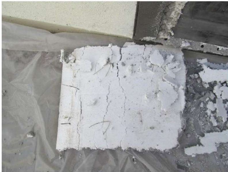
May 13, 2019, Disc IT1, Photograph 116, JBF, Building B, 1/2-inch-thick EPS insulation installed over OSB sheathing does not incorporate vertical grooves.
