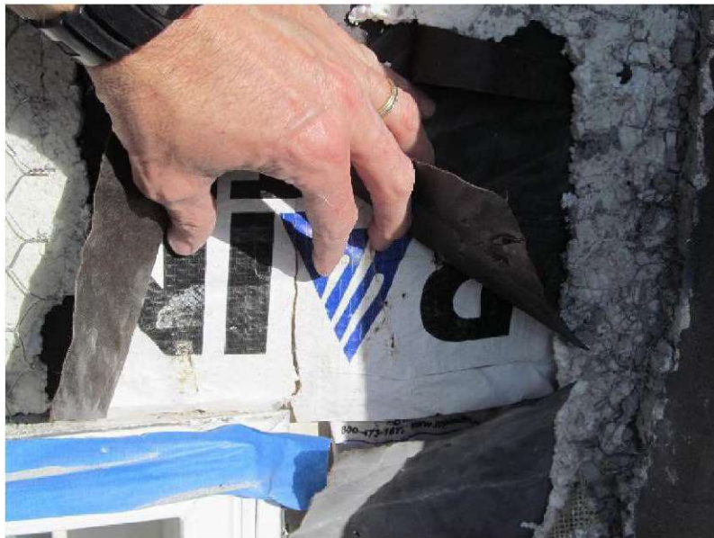
March 9, 2021, Disc IT5, Photograph 178, JIF, Building B, one layer of WRB over sheathing.
