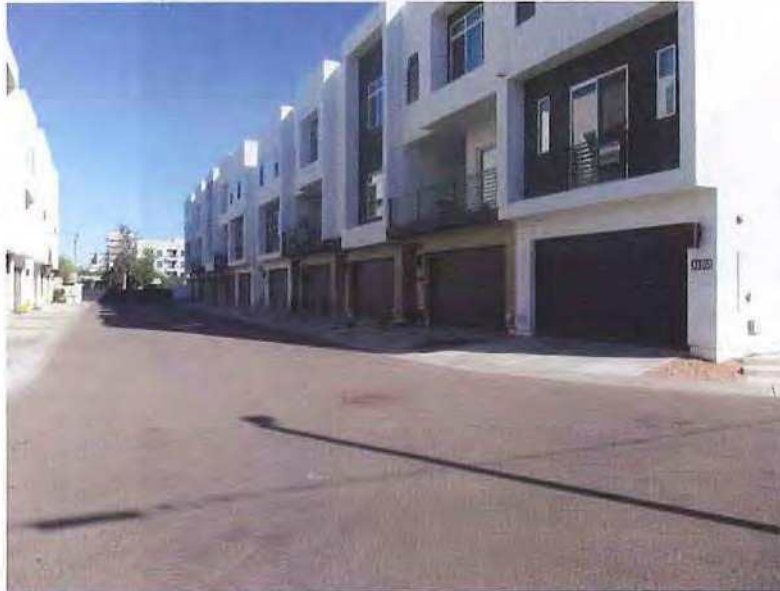
December 19, 2018, Photo 14, OBS1, JBF, overview of the elevation showing limited panel size available for LFRS.
