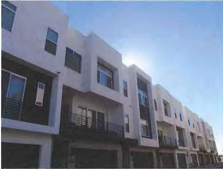
December 19, 2018, Disc OBS1, Photograph 5, JBF, west elevation of Buildings C and D, no control/movement joints provided.
