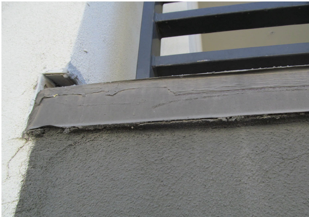
Deck metal properly installed over stucco
